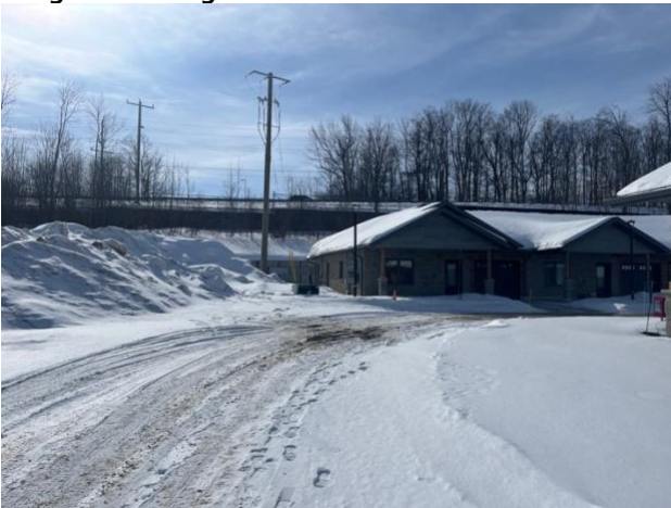
Image 2: Looking South from Site Towards 10 th Street East Retaining Wall
