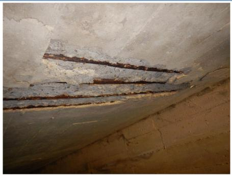
View of severe soffit spall with exposed corroded reinforcing and adjacent delamination.
