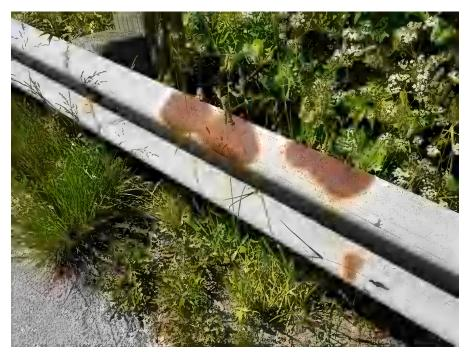
View of minor barrier corrosion.
