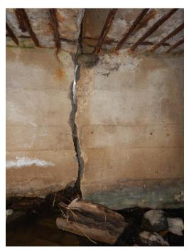
View of full height north abutment 50mm crack.
