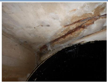
View of spall with exposed and corroded reinforcing steel above west barrel.
