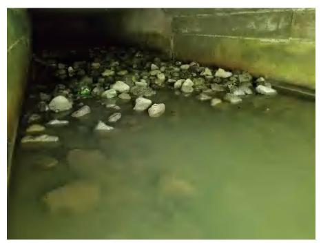
View of sediment buildup in barrel.
