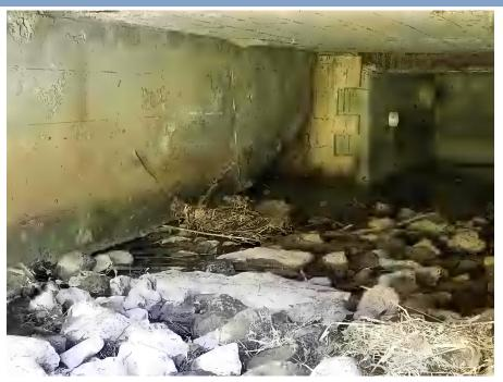
View of severely deteriorated north abutment.
