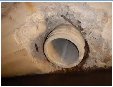
View of spall and exposed reinforcing in the east abutment at the storm drain penetration.
