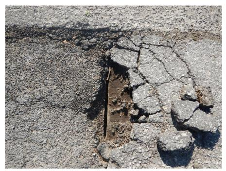
View of wearing surface pothole showing a steel plate support.
