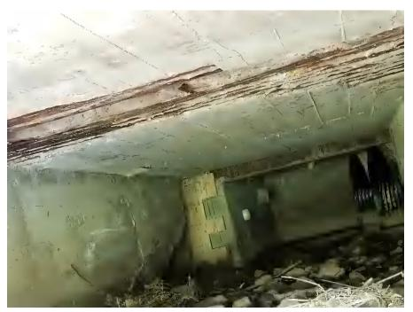
View of severe soffit spall near midspan.
