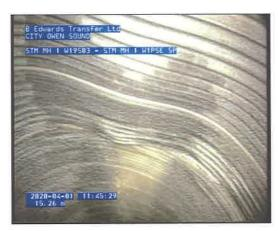
Photo: 4\_1A 15.26m, Deformed, 5 % changed
