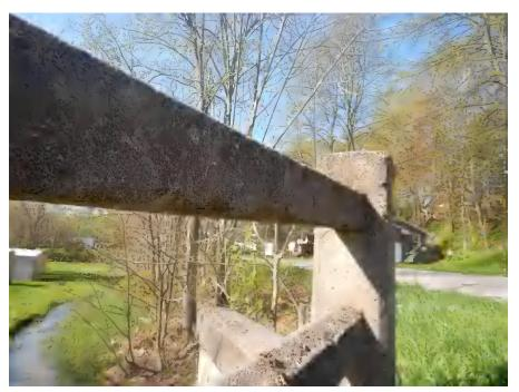
Spalling of barrier rail.
