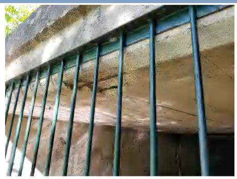
View of severe spall at inlet.
