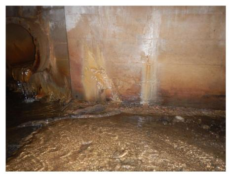
View of west abutment efflorescence.
