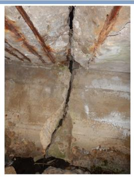
View of full height south abutment 50mm crack.
