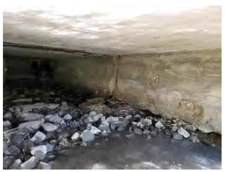
View of severe crack in south abutment wall.
