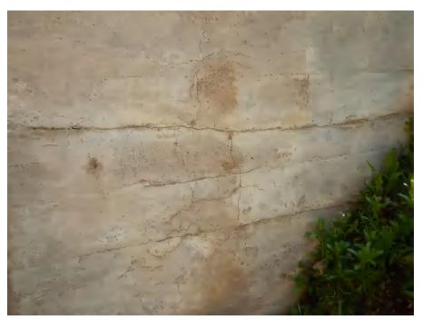
View of map cracking on southeast wingwall.
