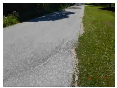
View of alligator cracking.
