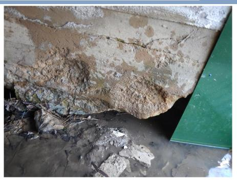
View of abutment undermining and scour at southwest corner.
