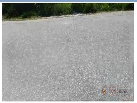
View of transverse crack in southeast approach.
