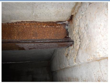
View of outlet cistern steel beam corrosion.
