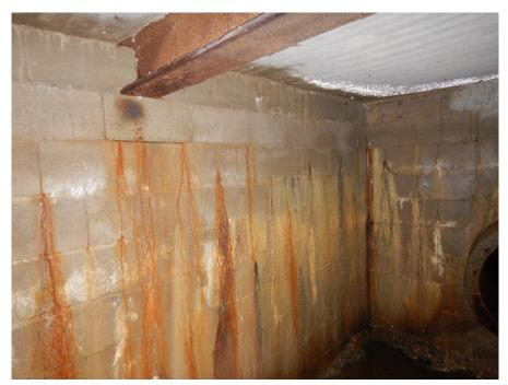
View of outlet cistern block wall efflorescence.
