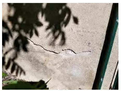
View of delamination on northwest wingwall.
