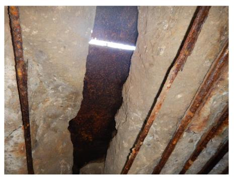
View of 175mm soffit crack near mid span. (visible daylight through deck)
