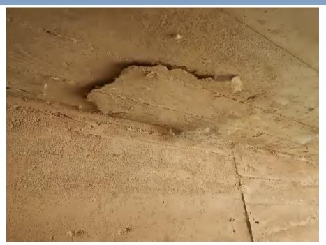
View of delamination on soffit near east abutment interface.
