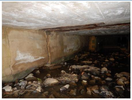
View of typical undermining at north abutment base.
