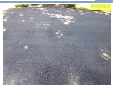
View of narrow crack in deck wearing surface.
