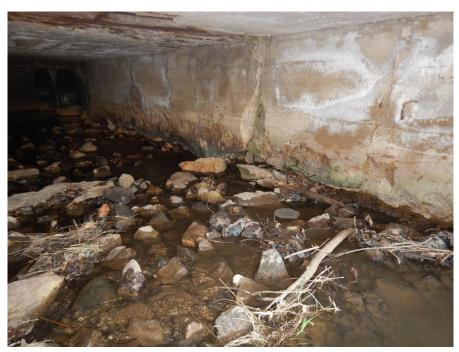
View of typical undermining at south abutment base.
