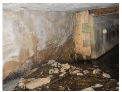
View of deteriorated and collapsed north abutment.
