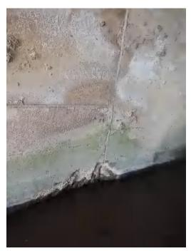
West abutment severe spall.
