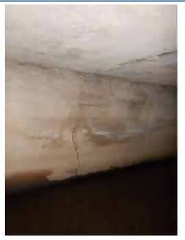
View of narrow crack in west abutment.
