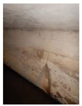
View of narrow crack in east abutment.
