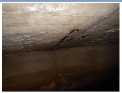
View of typical soffit spall and delamination with exposed corroded reinforcing.
