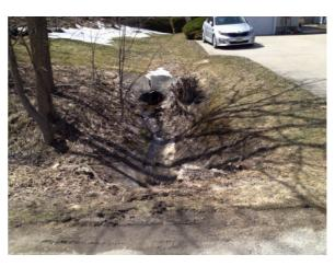
Photo 19, Upstream of culvert, concrete then buried pipe
