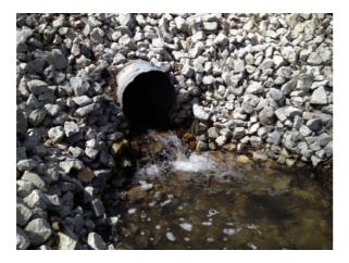
Photo 18: Perched culvert outlet at site 10, Fish Barrier
