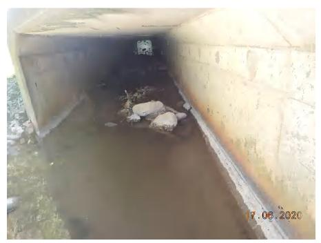
View of debris buildup in barrel.
