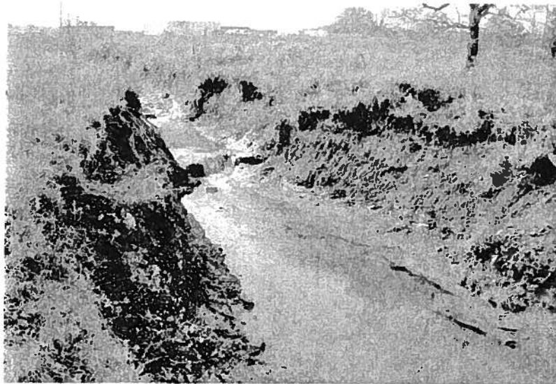
looking upstream over the cross-section location
