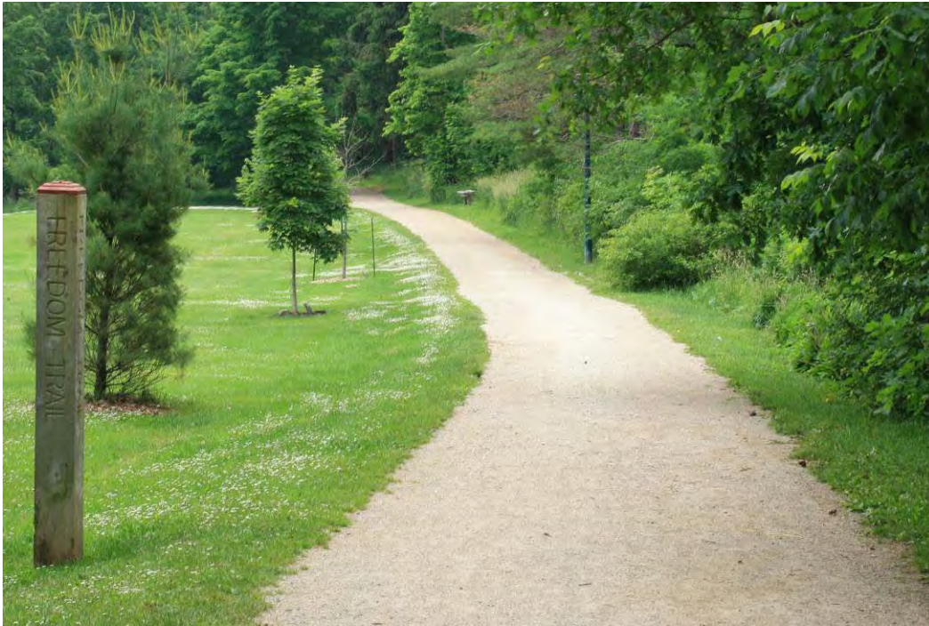
This photo represents one of the most popular trail routes in Owen Sound. This stone dust section of the Freedom trail in Harrison Park is an example of a multi-use surface for trail design. This material is an adequate trail base in areas with low erosion risk.
