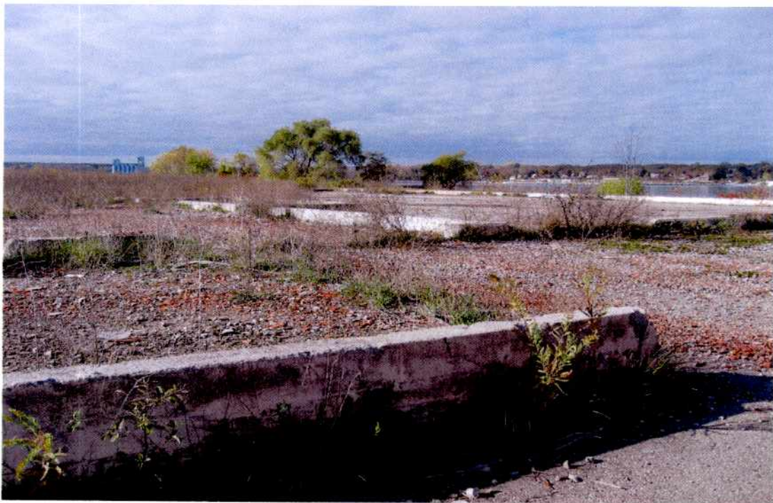
VIEW OF SUBJECT SITE, FACING SOUTHWEST (OCTOBER 23, 2006)
