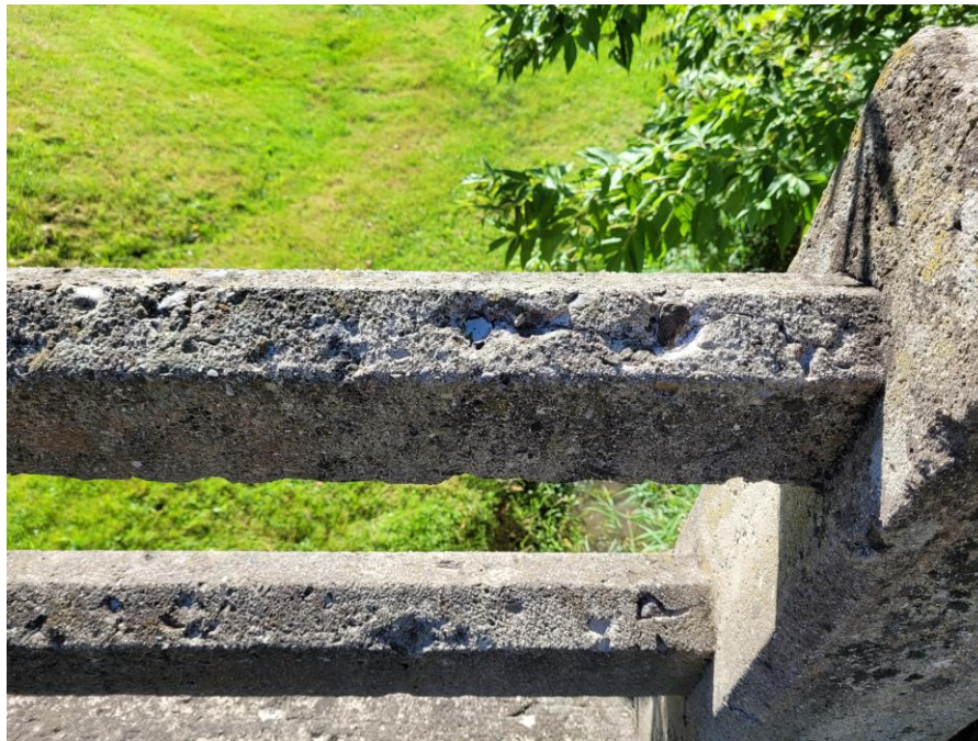
Spalling of barrier rail.
