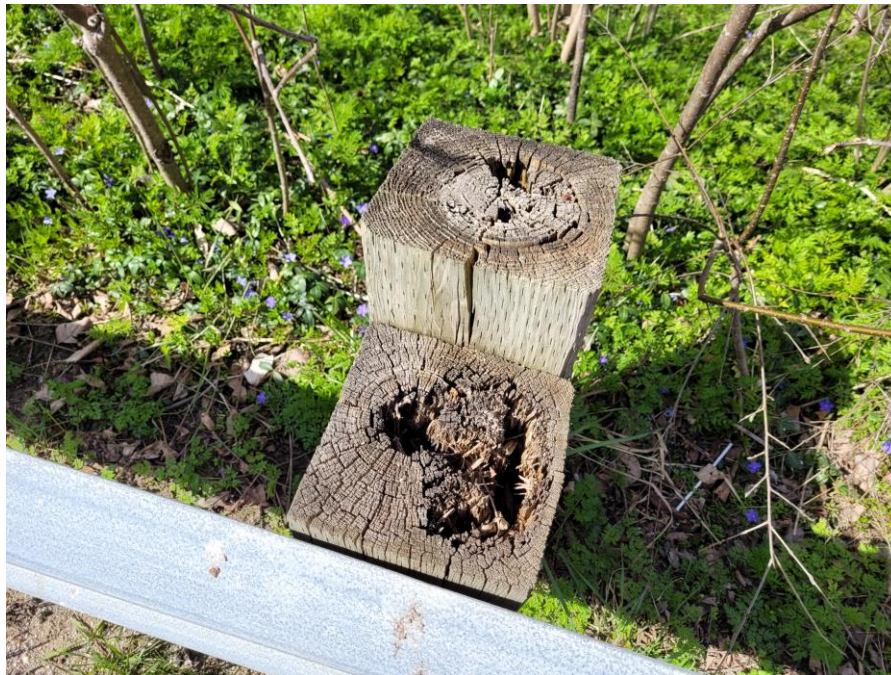
View of barrier post rot.
