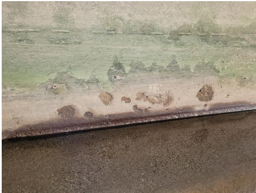
View of a spall at the base of the east abutment.
