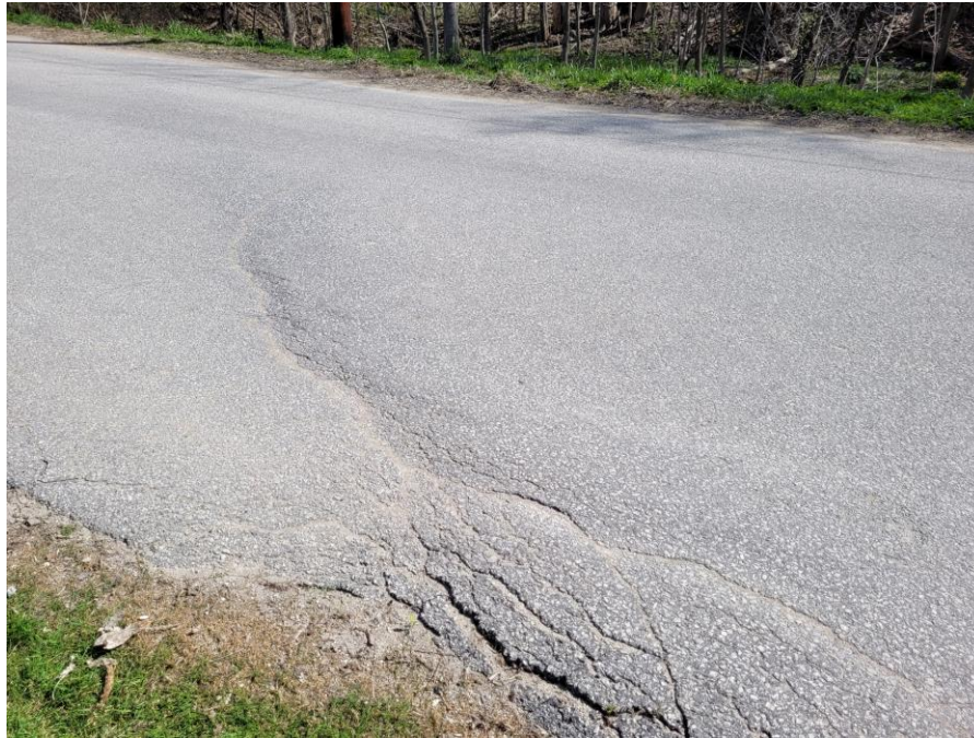
View of alligator cracking.
