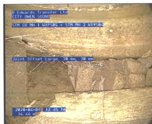
Photo: 5_10A 34.44m, Joint Offset Large, 30 mm, 30 mm
