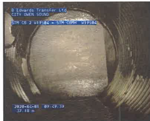
Photo: 2_3A 37.18m, Surface Roughness Increased Unknown, from 3 o'clock, to 8 o'clock
