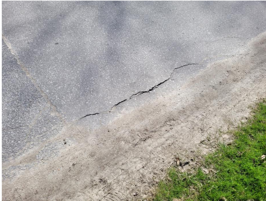
View of asphalt cracking along northwest approach.
