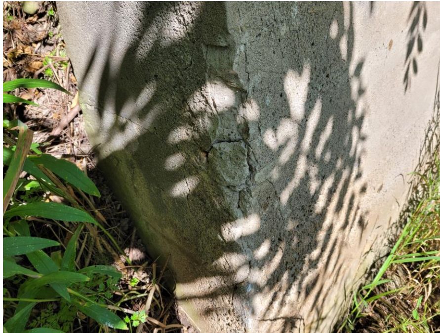
View of delamination on southwest wingwall.
