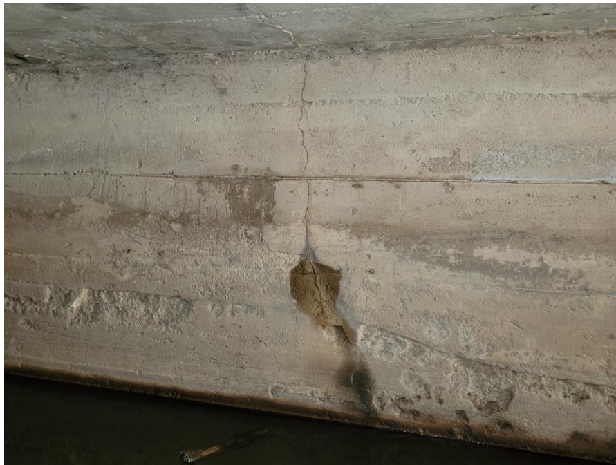
View of narrow crack in east abutment.
