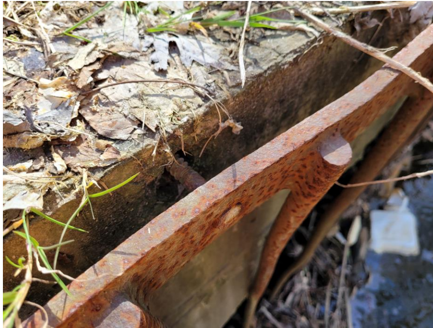
View of gate anchor being pulled from concrete.
