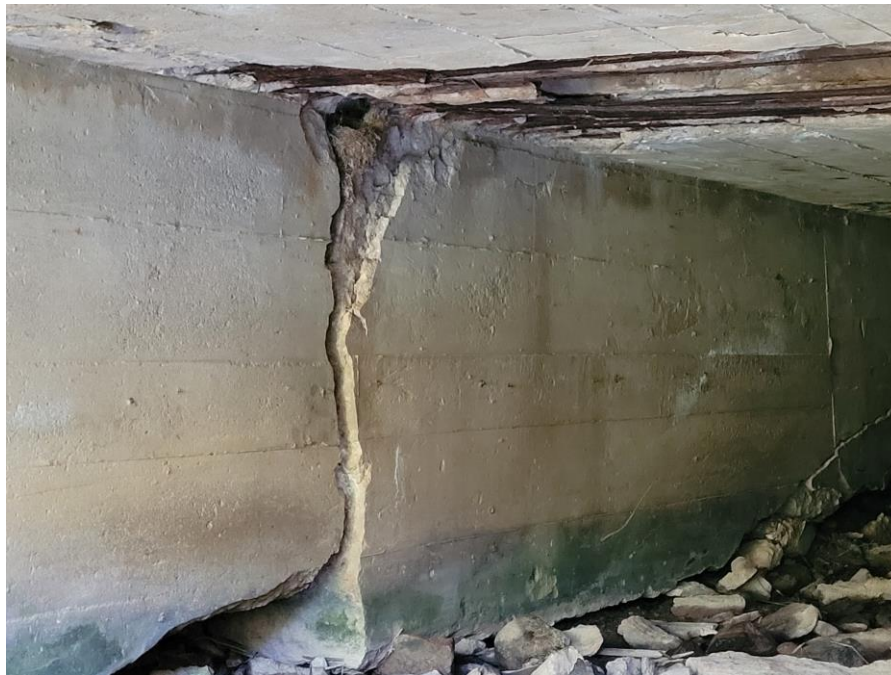
View of severe crack in north abutment wall.
