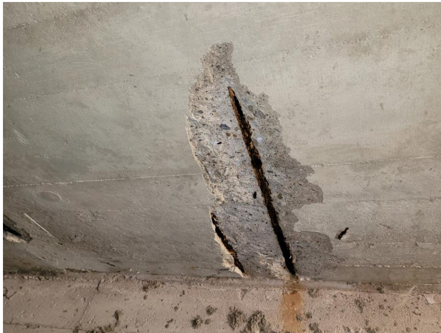
View of severe soffit delamination above storm drain.
