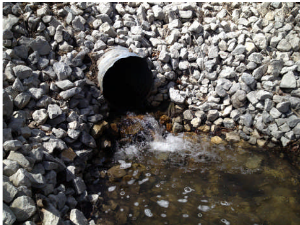
Photo 18: Perched culvert outlet at site 10, Fish Barrier
