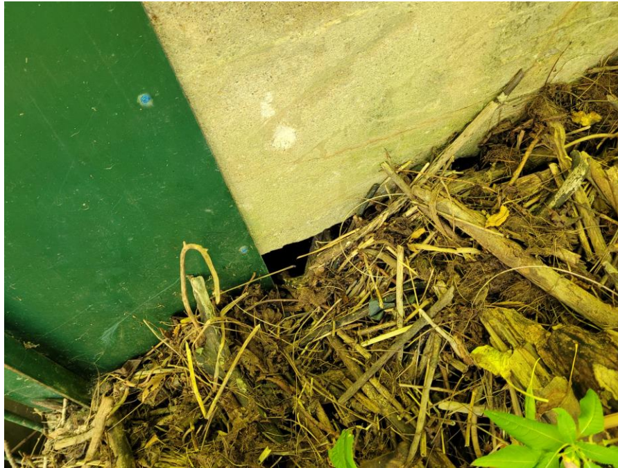
View of southwest wingwall undermining.
