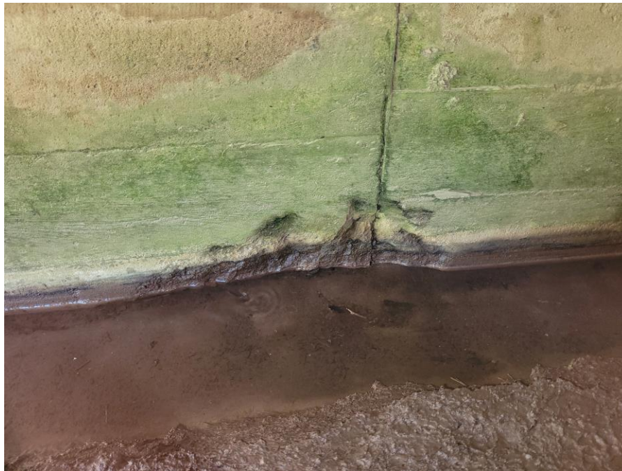
West abutment severe spall.
