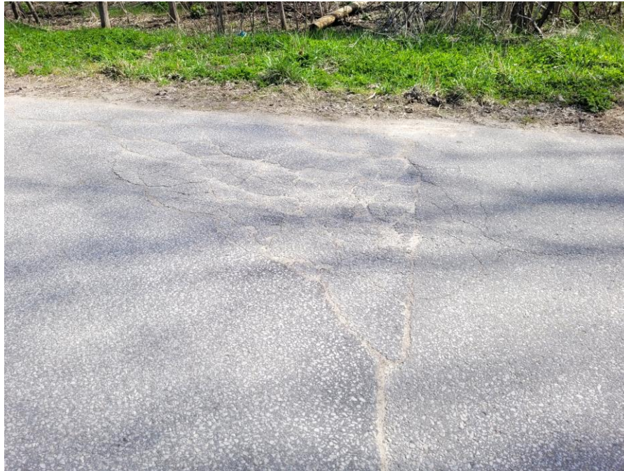
View of alligator cracking near southwest.
