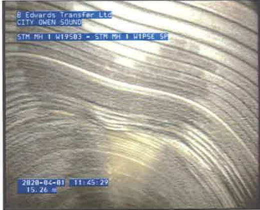
Photo: 4_1A 15.26m, Deformed, 5 % changed
