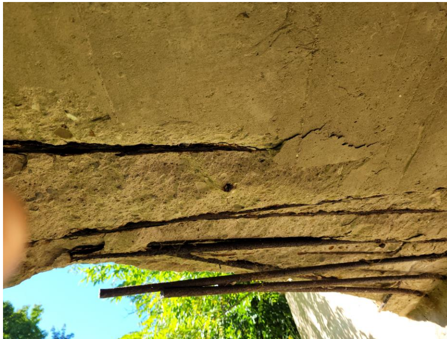
View of exterior soffit with severe spalling and exposed corroded rebar.
