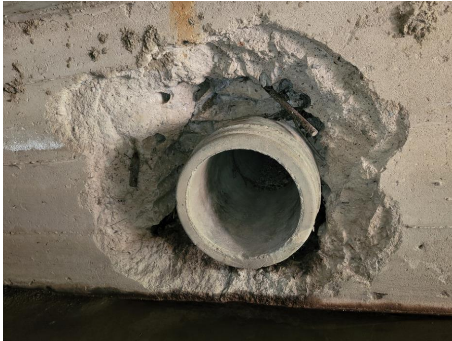
View of spall and exposed reinforcing in the east abutment at the storm drain penetration.
