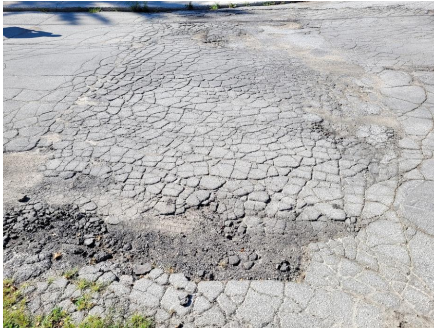
View of wearing surface with map and alligator cracking.
