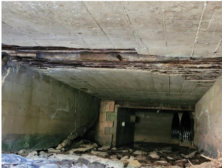
View of spall near midspan.
