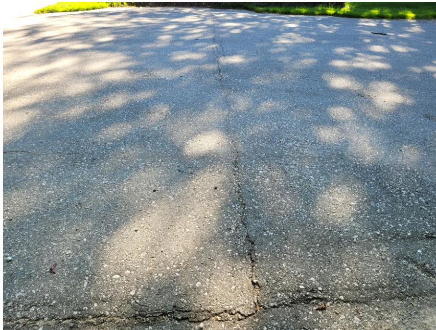
View of narrow crack in wearing surface.
