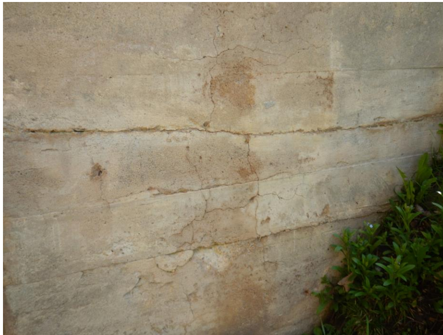
View of map cracking on southeast wingwall.
