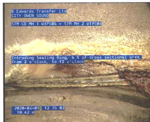
Photo: 5_3A 10.62m, Intruding Sealing Ring, 5 % of cross sectional area, from 2 o'clock, to 12 o'clock
