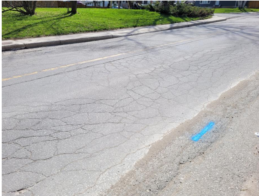
View of wearing surface alligator cracking.
