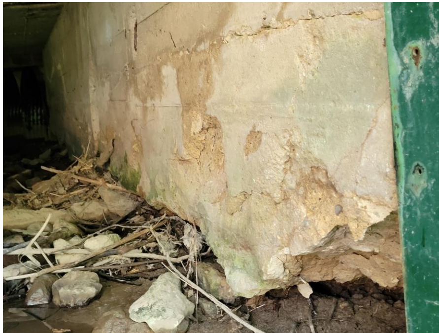
View of south abutment undermining.
