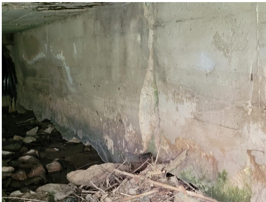
View of severe crack in south abutment wall.
