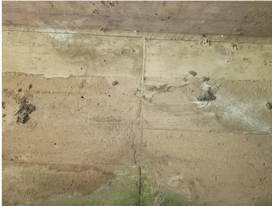
View of narrow crack in west abutment.
