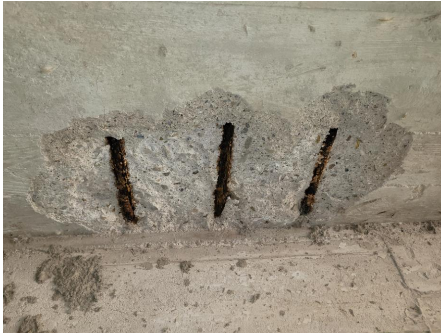
View of spall on soffit near east abutment interface.
