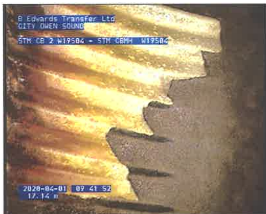
Photo: 2_1A 17.14m, Surface Corrosion Metal Pipe, from 5 o'clock, to 8 o'clock
