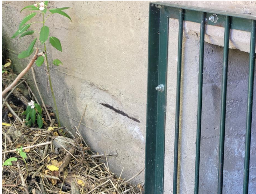
View of spall on northwest wingwall.
