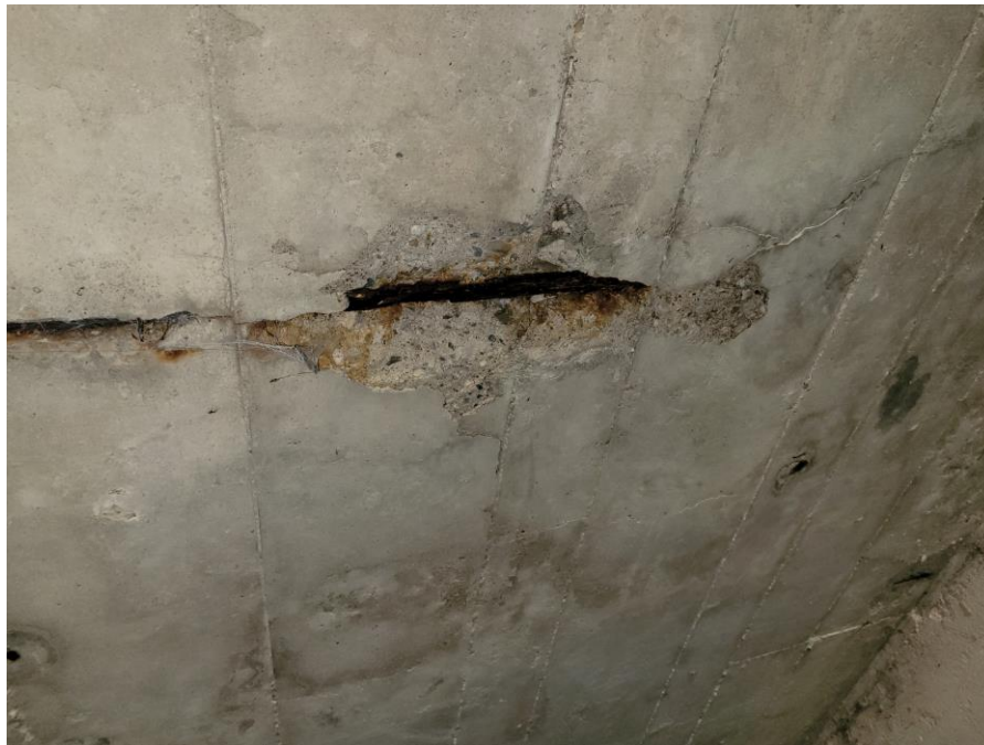
View of small soffit delamination following transverse crack.
