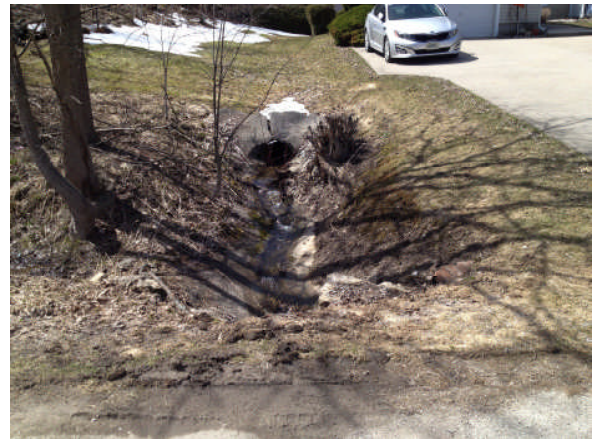
Photo 19, Upstream of culvert, concrete then buried pipe
