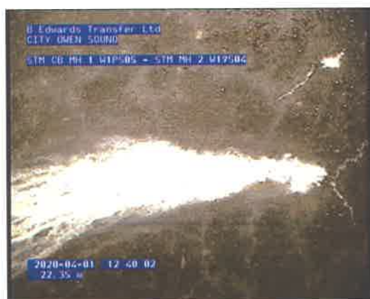
Photo: 5_6A 16.15m, Crack Multiple, from 11 o'clock, to 2 o'clock, 1 mm defective, 1 mm intrusion, Start
