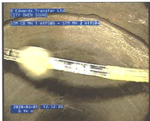
Photo: 5_1A 8.96m, Intruding Sealing Ring, 40 % of cross sectional area, from 3 o'clock, to 10 o'clock
