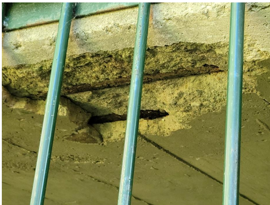
View of severe spall at inlet.
