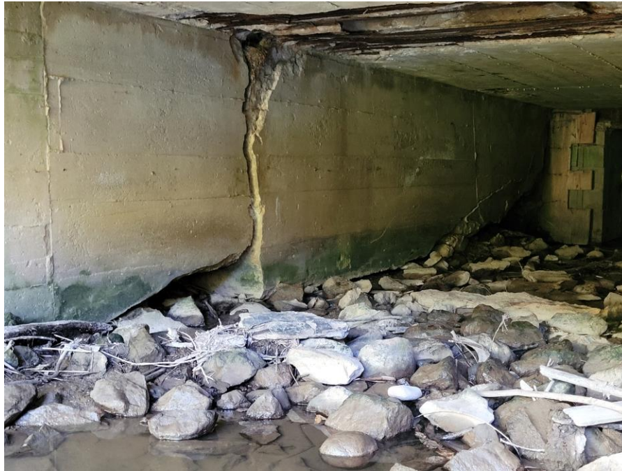
View of north abutment undermining.
