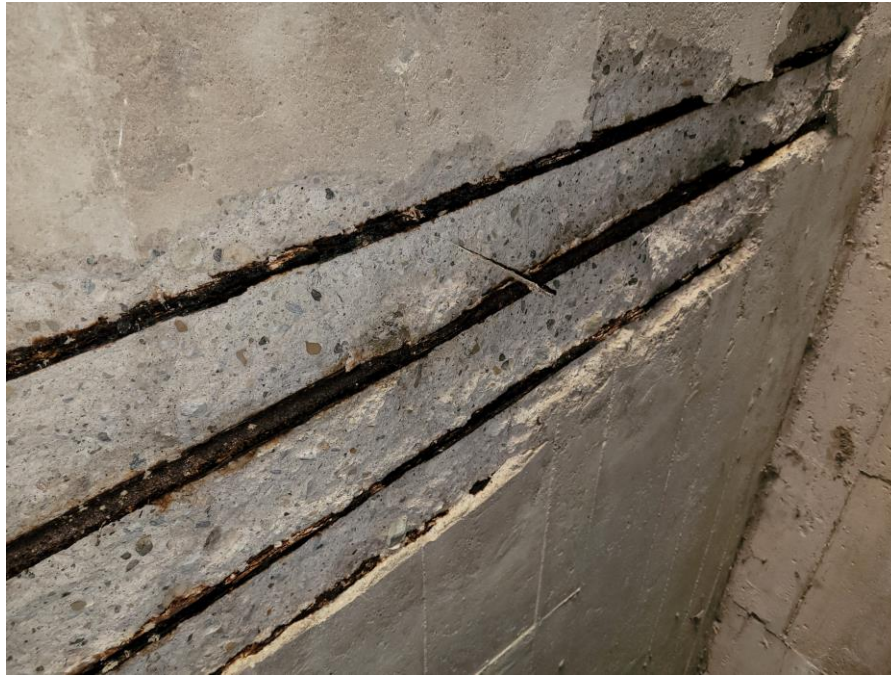
View of severe soffit spall with exposed corroded reinforcing and adjacent delamination.
