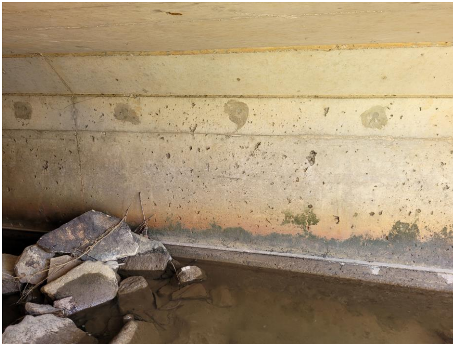
Minor honeycombing on abutment wall.
