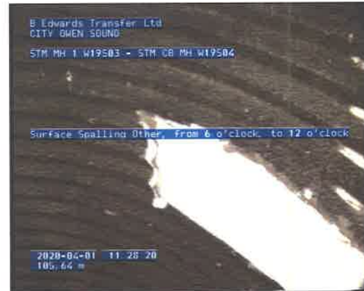
Photo: 3_7A 105.64m, Surface Spalling Other, from 6 o'clock, to 12 o'clock
