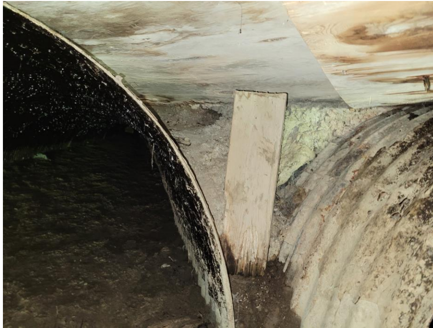
View of deteriorated headwall.
