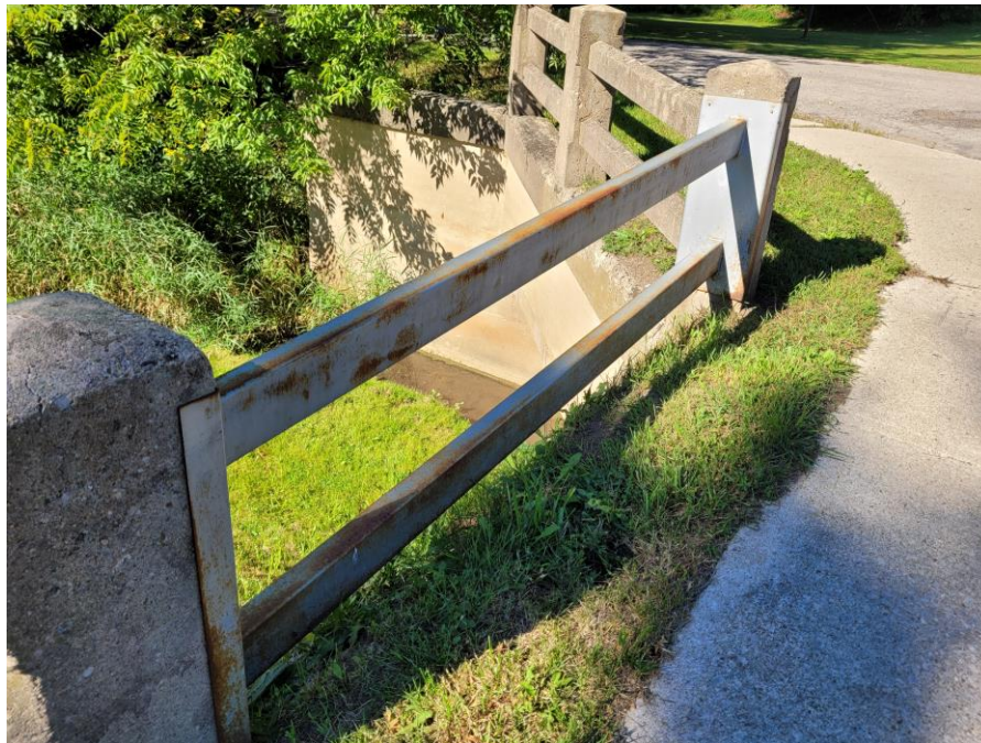
View of barrier rail repairs with moderate corrosion.
