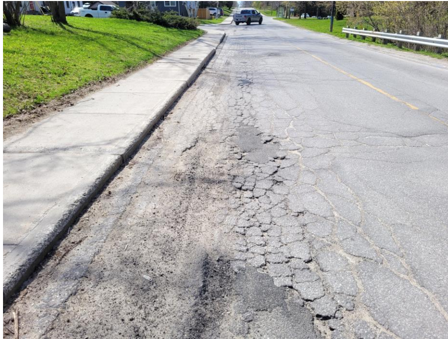
View of wearing surface potholes.
