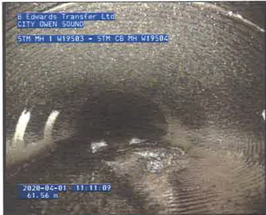
Photo: 3_3A 61.56m, Surface Spalling Other, from 9 o'clock, to 6 o'clock
