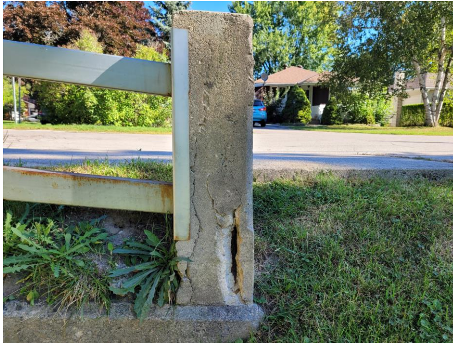
View of east barrier post with spalling.
