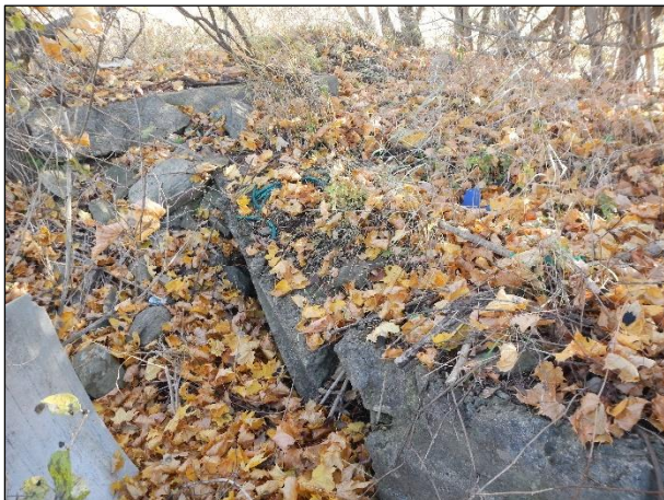
Image 3: Disturbed Area – Concrete Slabs (Facing SE)
