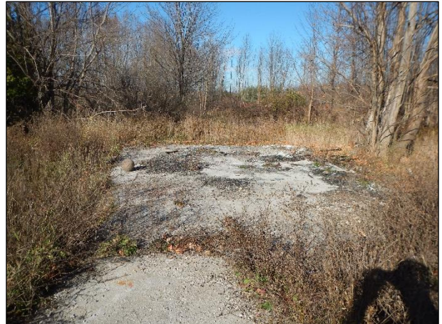
Image 12: Disturbed Area – Existing Concrete Pad (Facing N)
