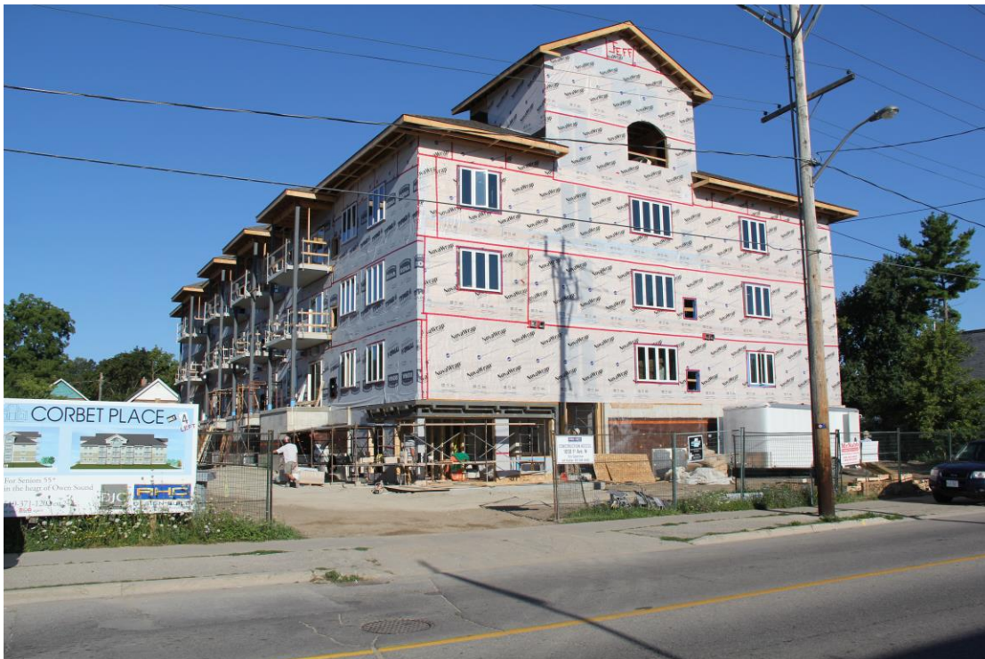
Corbet Place (1050 1 st Ave W) under construction
