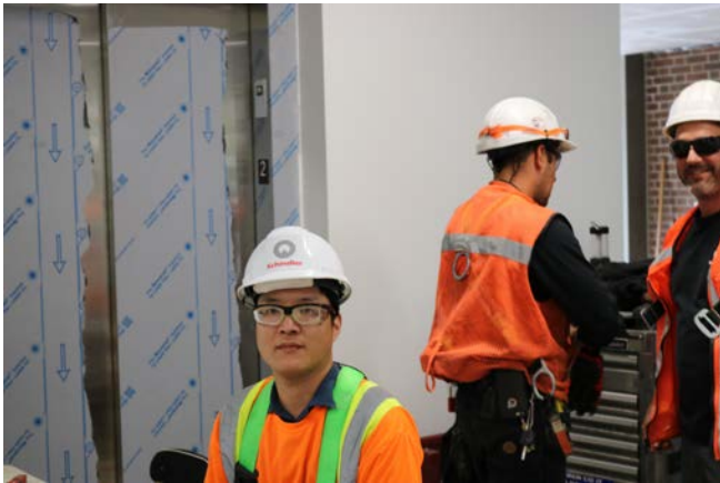
On site contractors finishing the accessible elevator installation
