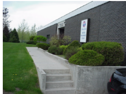
(Richard H. Neath Water Treatment Plant- front entrance)
